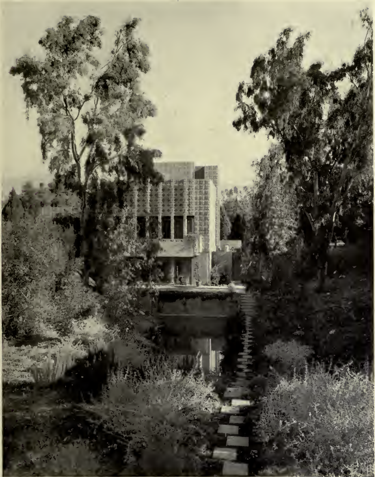
"La Miniatura," a residence in Pasadena, California, built in 1923 of textile-blocks, is typical of a new type of reinforced concrete construction. The square lines and terraced roofs, which have inspired recent European architecture, have for many years been typical of Frank Lloyd Wright's Prairie Architecture.
